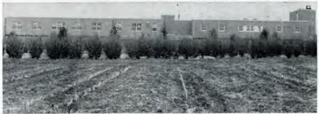
Addition to Home nearly completed
