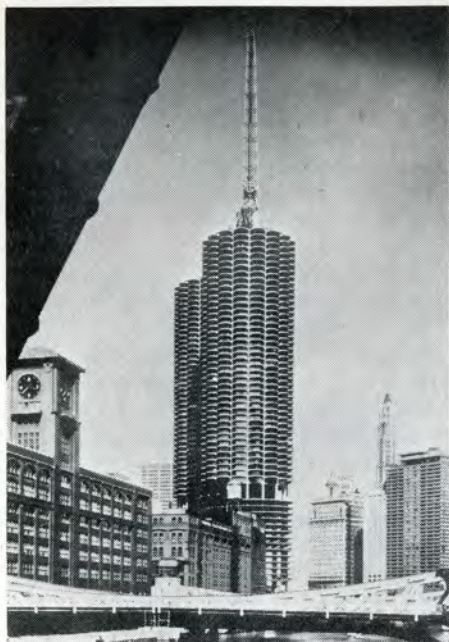
Marina City's towers framed by the Merchandise Mart in the left foreground and the Wrigley Building in the background at right.
