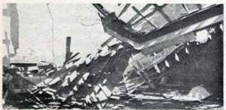
Lodge Room after Tornado, north view.
