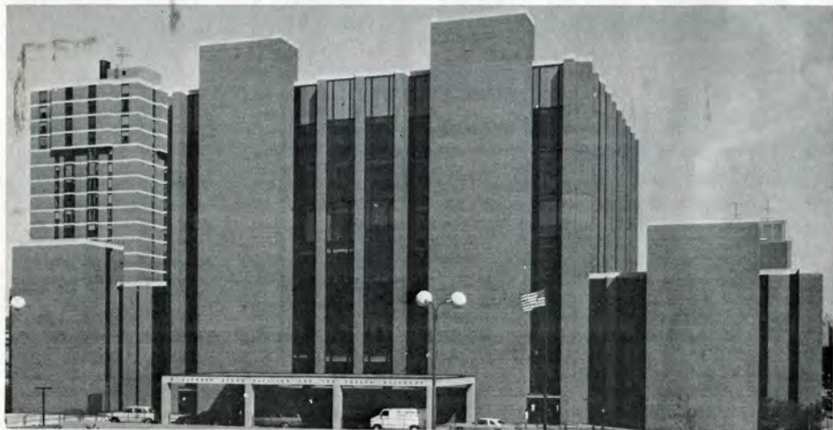
W. Clement Stone Pavilion for the Health Sciences, Illinois Masonic Medical Center
