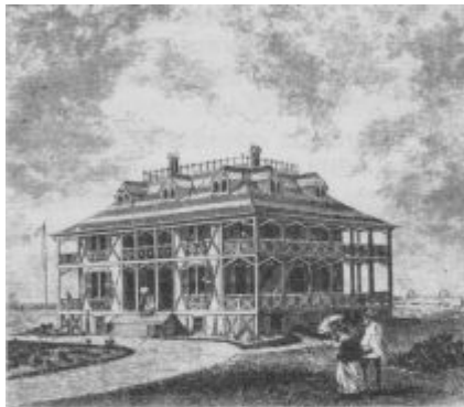
Summer cottage at Long Beach, New Jersey, built during President Grant's first term, serves to illustrate what the Weekly considered "a very tasteful and elegant bit of summer architecture."
